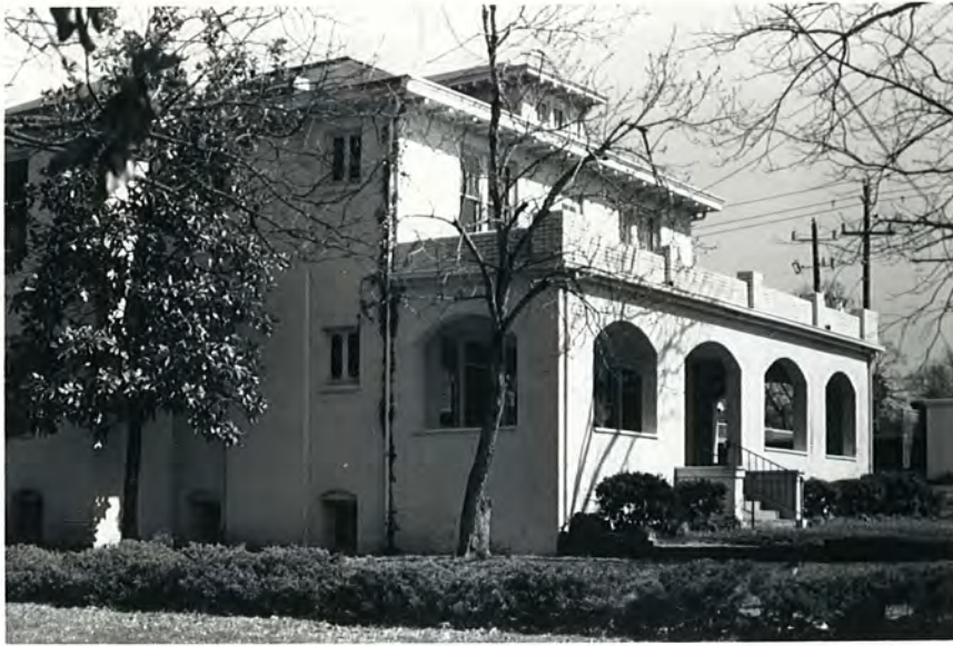
Plate 28. Hurley House, Looking North.
