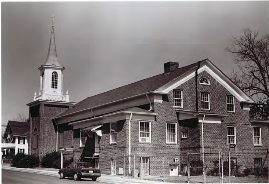
Plate 34. First Presbyterian Church, Rear and West Elevations, Looking North.
