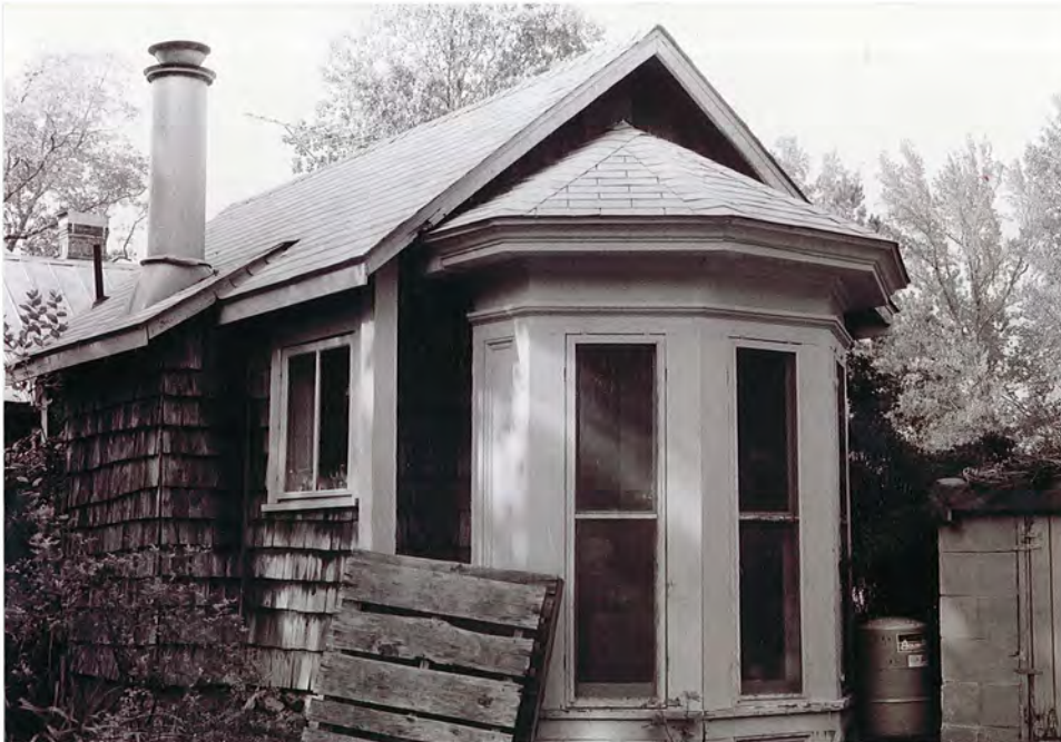
Plate 60. Neal Clark House, Studio (Former Woodshed/Powerhouse).
