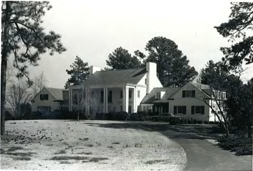
Plate 21. Paul Russell House, House and Setting, Looking Southeast.
