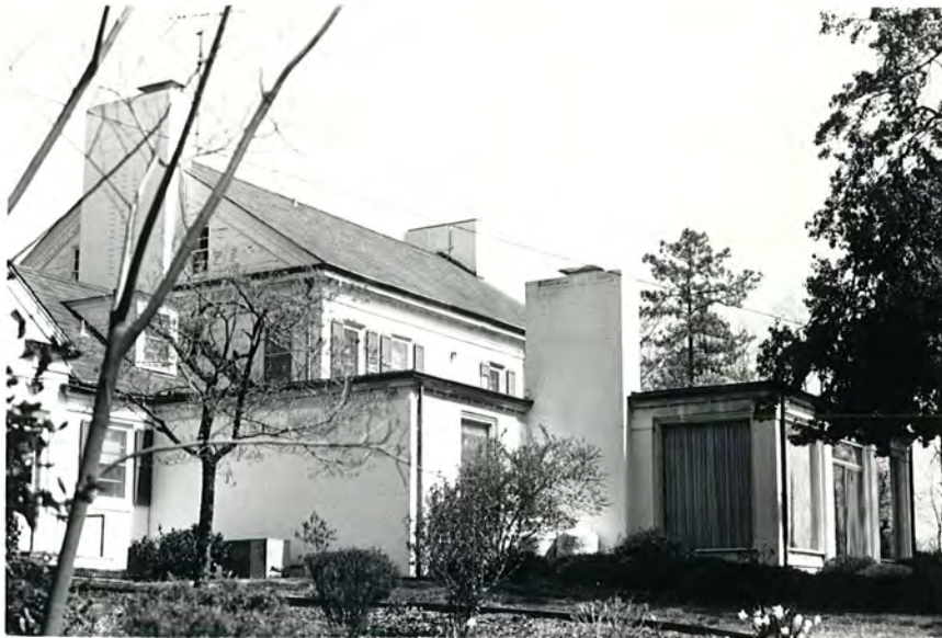
Plate 23. Paul Russell House, Rear Elevation, Looking Northeast.
