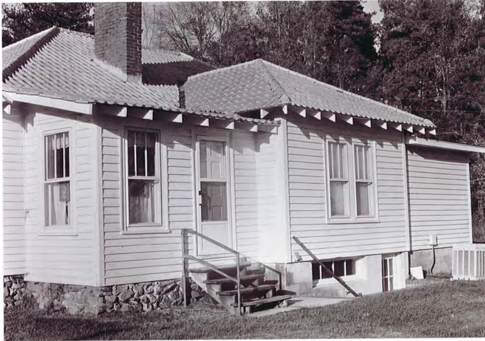
Plate 63. Laughlin-Saunders House, Rear Elevation, Looking North.
