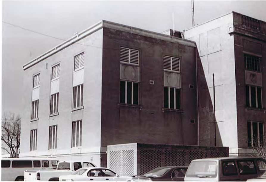
Plate 3. Montgomery County Courthouse, Rear Addition, Looking Northwest.
