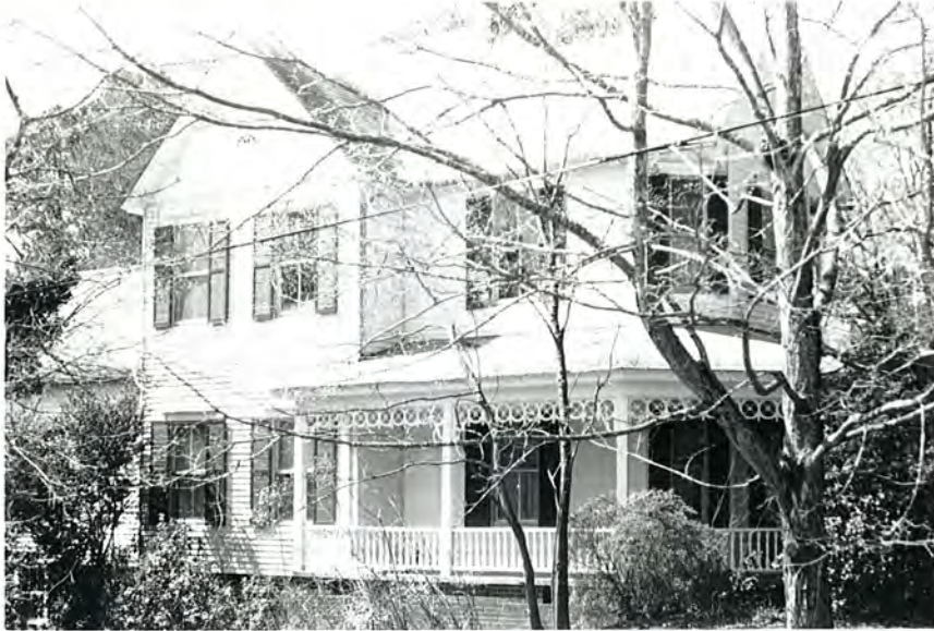
Plate 13. Robert Terrell Poole House, East Elevation, Looking West.
