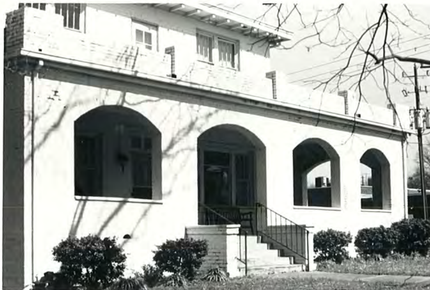
Plate 29. Hurley House, Front Porch.
