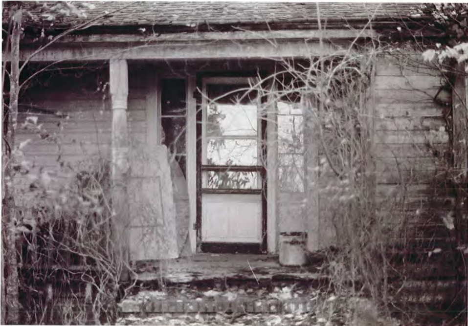
Plate 41. Wooley-Saunders House, Main Doorway, Looking South.
