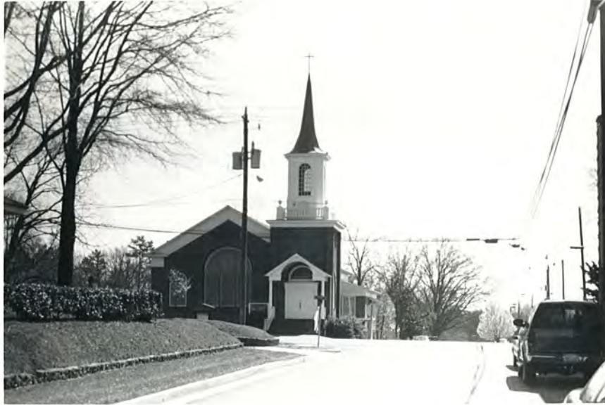
Plate 33. First Presbyterian Church, Looking South.
