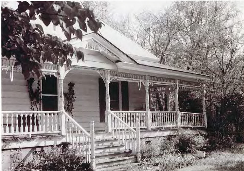
Plate 53. Neal Clark House, Porch, Looking Southeast.
