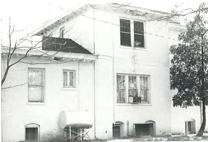
Plate 30. Hurley House, West Elevation, Looking East.
