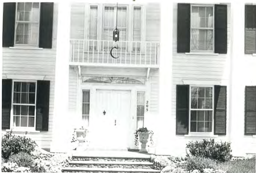
Plate 9. Capel Family House, Entrance Detail.
